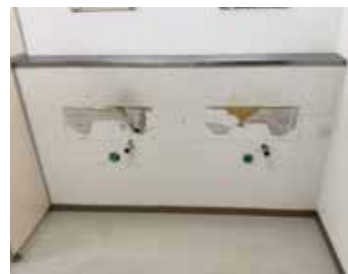
②既存手洗い器撤去
